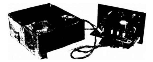
A simple two-tube transmitter and regenerative receiver believed to be used by the Viet Cong. The system is contained in a crude square container; it apparently operates on dry cell batteries.
